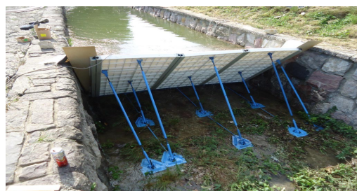
Fig. 6. Static test under real conditions of hydrostatic loading in canal
